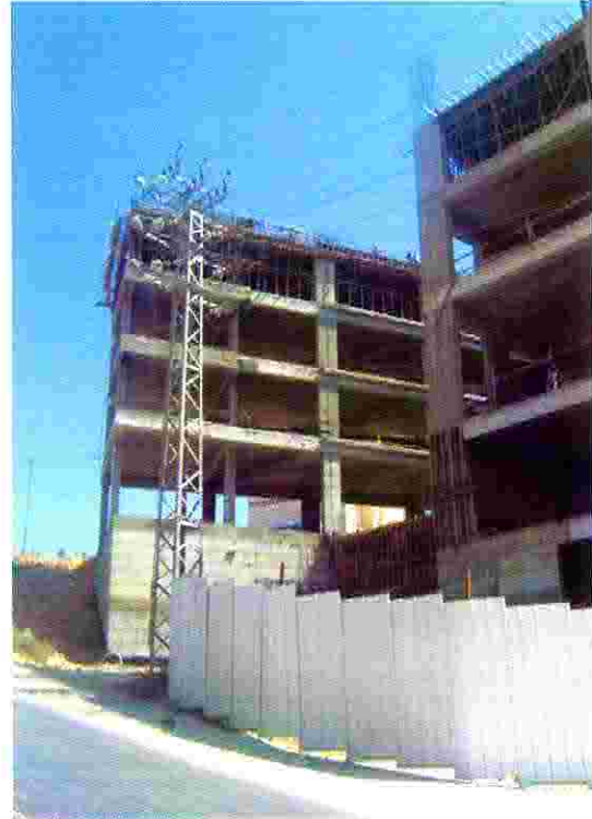
High Voltage Pillar
