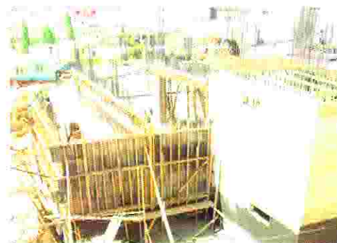
Ground Floor Southern wall
