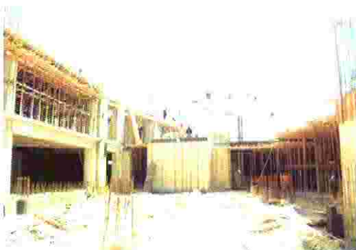
Ground Floor Slab for the Reception
